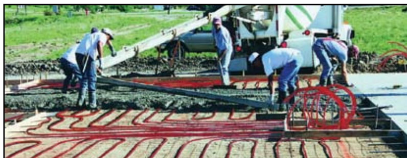
Figure 11.1 – Radiant Floor Heating Piping
