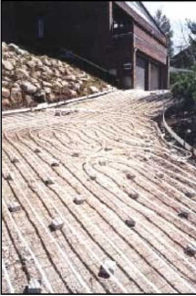
Figure 11.2 – Snow and Ice Melt Piping for a Driveway
