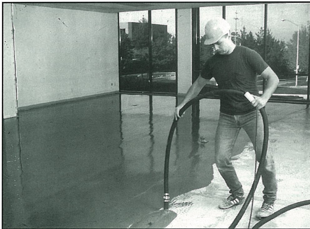
Fig. 3. Self-leveling floor toppings and underlayments are used to provide a smooth, level floor surface and to repair floors that have deteriorated, sagged, scaled, or become worn.
